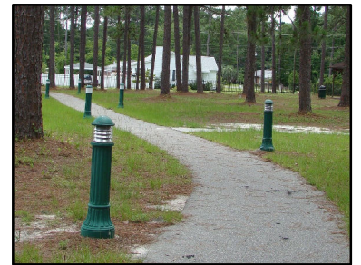
Bollards add subtle light limiting glare
