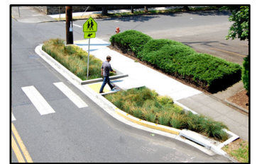
Crossing improvements at US 278 will increase safety and act as a gateway to local schools as well as other key community facilities
