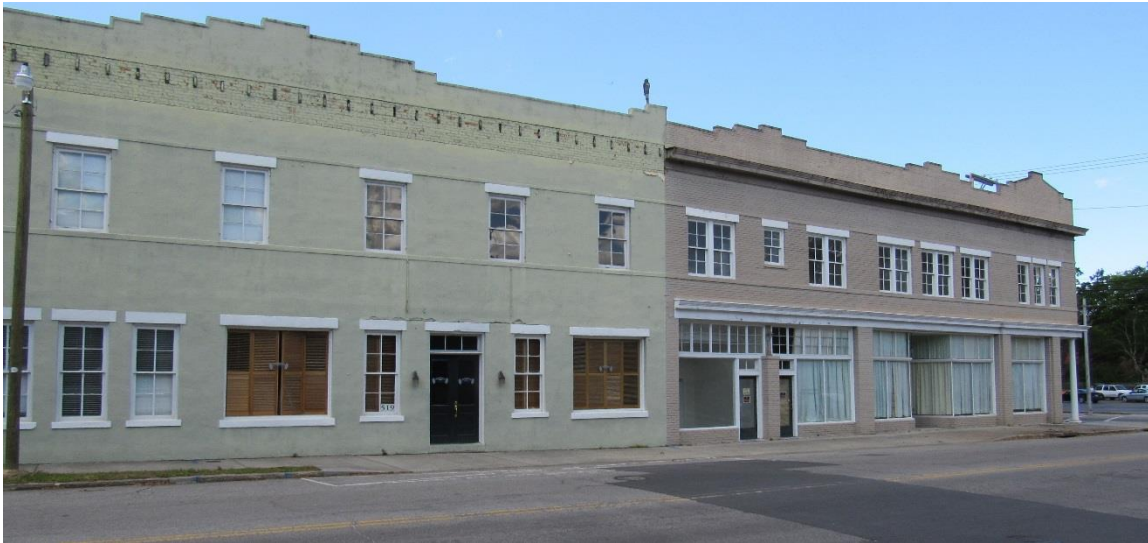
Former Hotel Building
