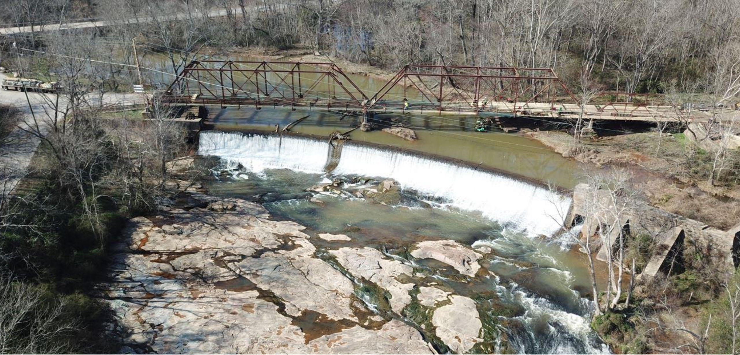
Glendale Historic Bridge before restoration
