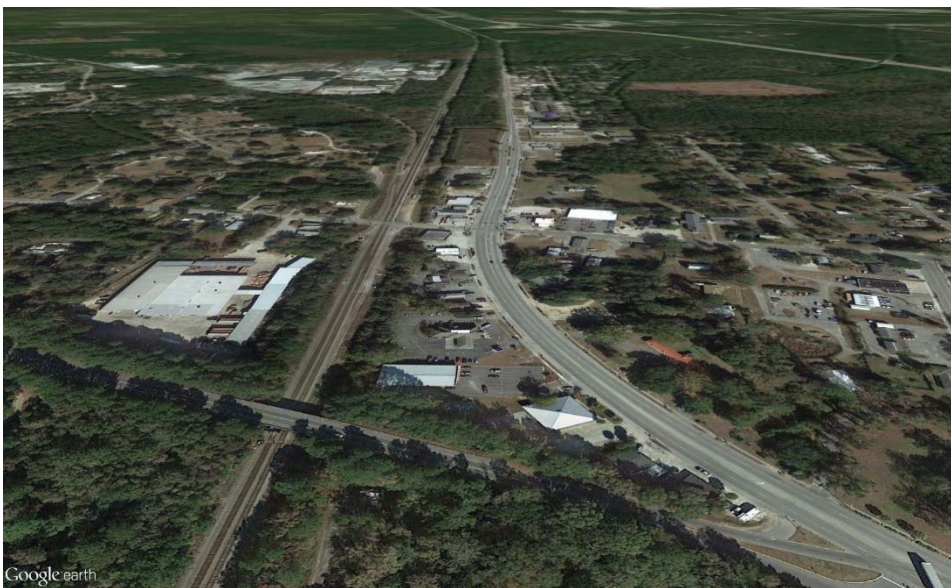
CSX Railroad and US 17 in Hardeeville
