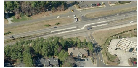
Directional Crossover (Left-Over)
